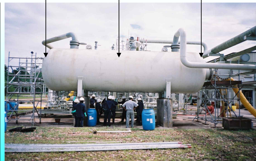
Fig. Separators of JB Process Plant showing different locations of radiation dose measurement. Sludge location (above).
