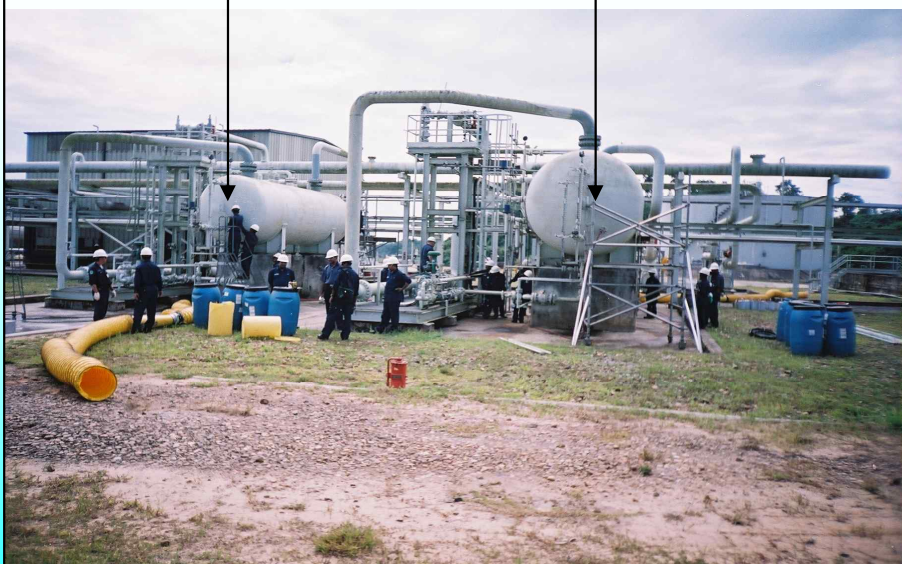
Fig. Separators of JB Process Plant showing different locations of radiation dose measurement. Sludge location (above).
