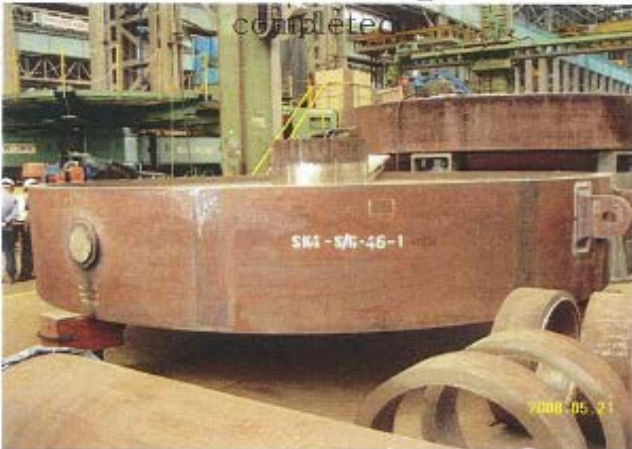
#4A : Tubesheet Cladding has been completed.
