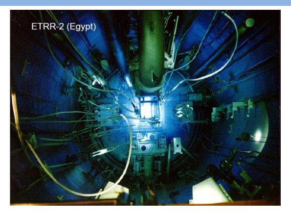
It houses the reactor core, reactor internal components, irradiation positions, beam tubes and connected to an auxiliary pool for spent fuel and radioactive material storage through transfer channel
